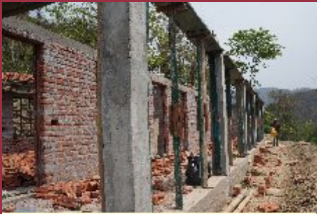
Construction at PS Bagwan
