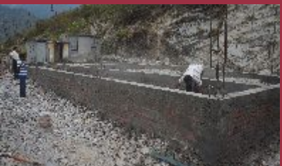
Construction underway at PS Mulya
