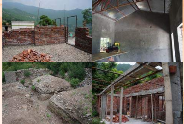
Schools under construction
